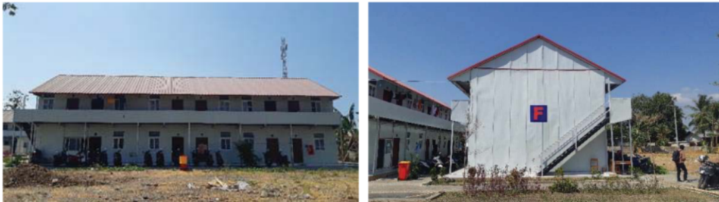
FIGURE 4. The dormitory is 2-storey constructed by lightweight steel frame construction
